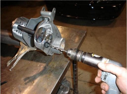
Mark the old lower perch  $\frac{3}{4}$ -inch from the back of each bolt hole and 1 1/8-inch from the top of each bolt hole. These will be your cut lines for removal .
