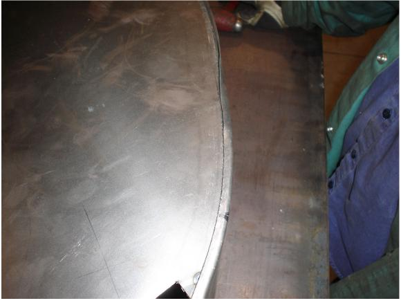
Work the locking seam over by hammering and working from one end of the tub to the other.
